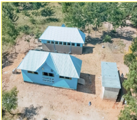
Aerial picture of the new & old toilet block
