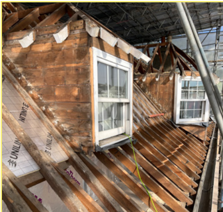
Rectory roof repairs in progress.
