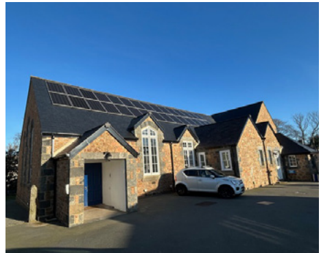
Parish Hall with solar panels
